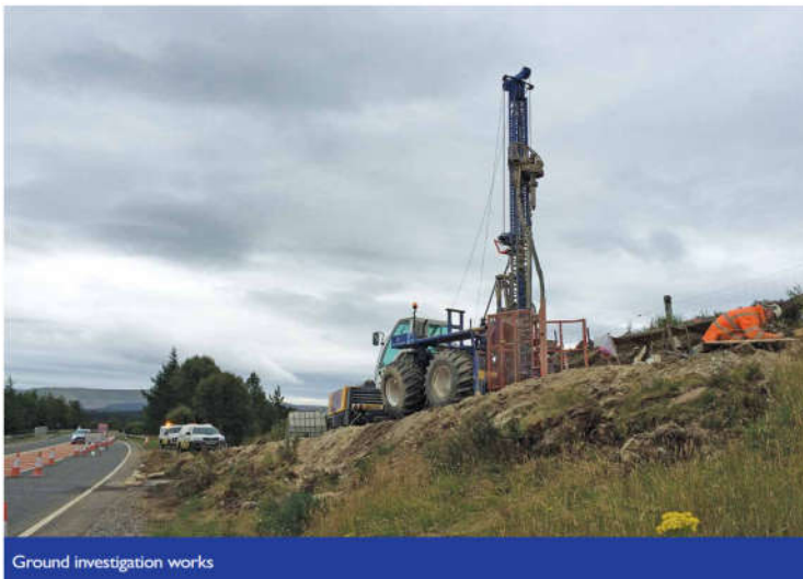
Ground investigation works
