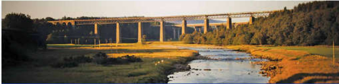
View of the Highland Main Line railway and existing A9 looking north-west, passing over the River Findhorn
