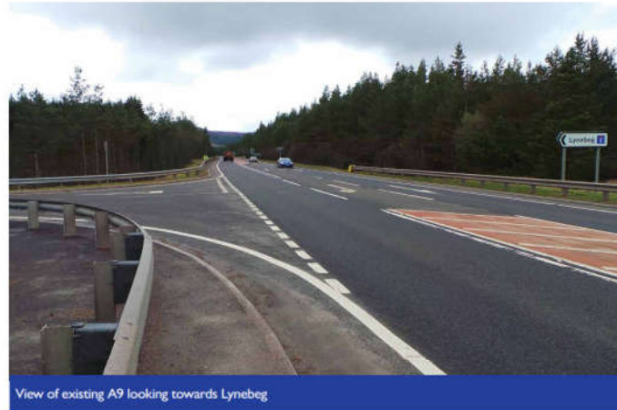
View of existing A9 looking towards Lynebeg
