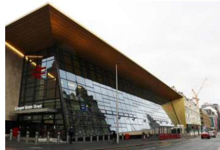
Glasgow Queen Street Station Improvements
