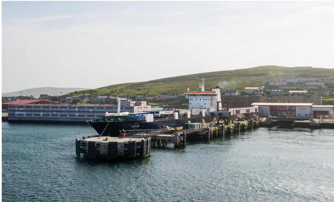
Figure 5: Lerwick Ferry Terminal
