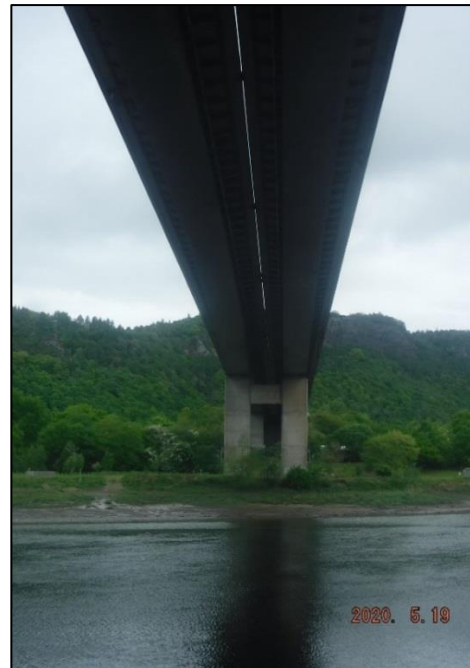
Figure 3. Pier 7 (looking north). Source: BEAR Scotland
