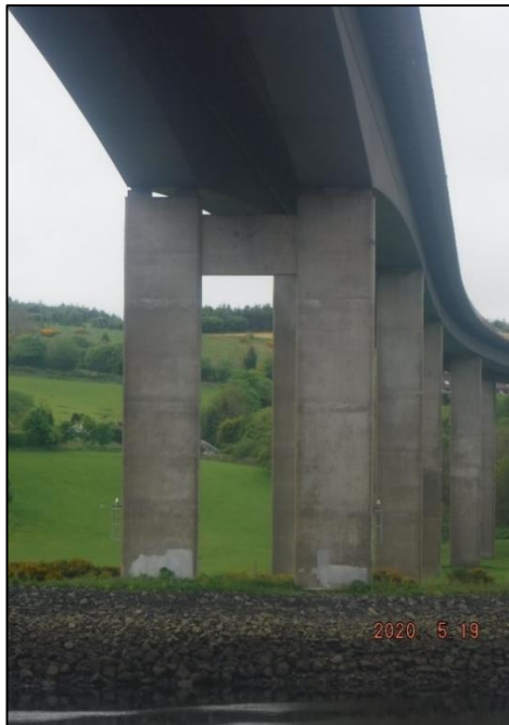
Figure 2. Pier 6 (looking south). Source: BEAR Scotland
