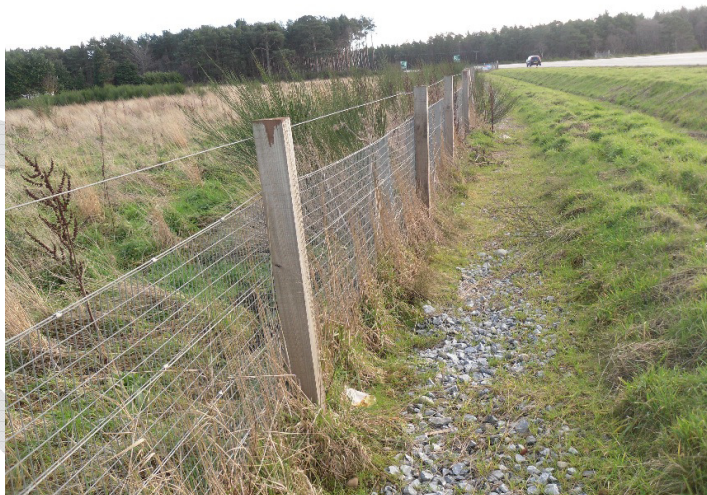
Figure 2 – filter drain with weed growth
