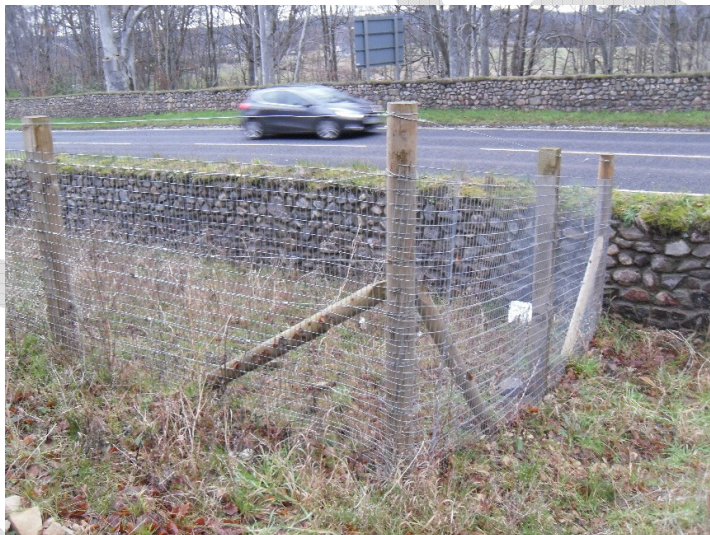
Figure 4 – installation of badger fencing
