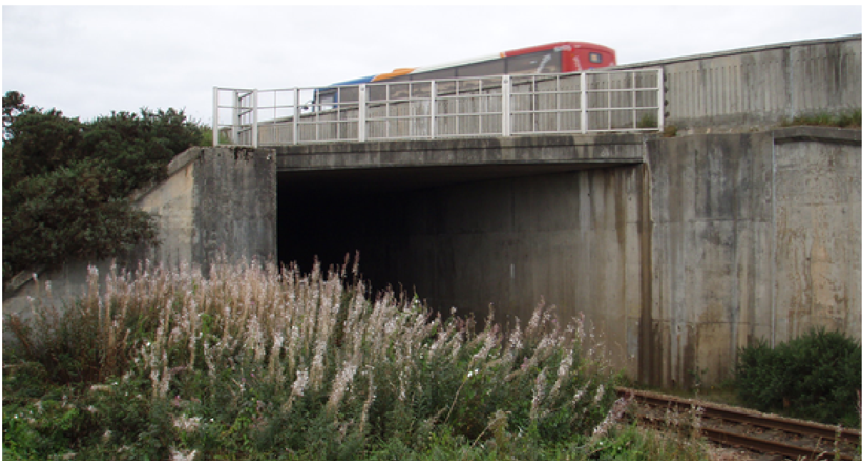
Photo 2.4: Existing Gollanfield Rail structure looking west (Reference No. A96 550)
