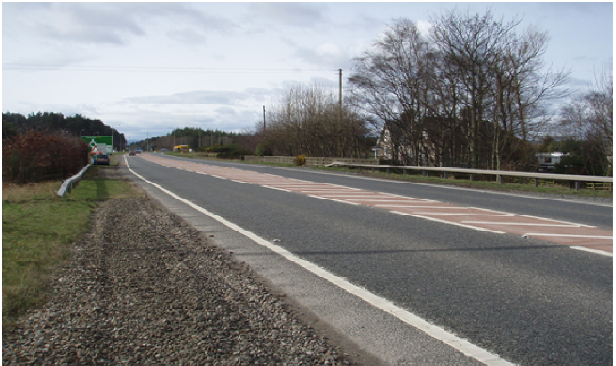
Photo 2.2: Existing drainage looking westbound on approach to the Airport Roundabout
