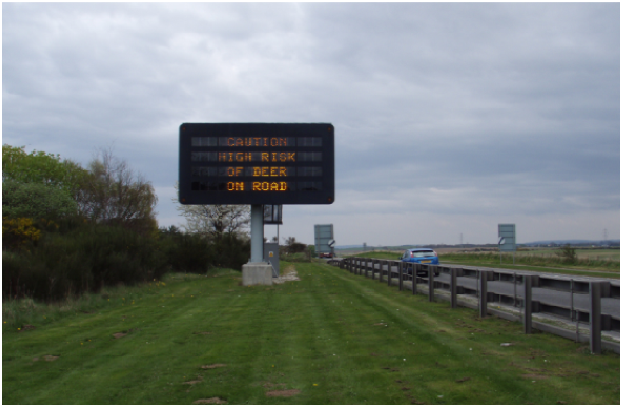
Photo 2.8: Existing VMS/A13 Nairn Sign Gantry (Reference No. A96 528 G51)
