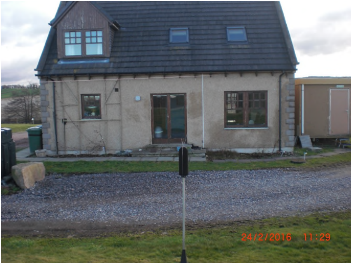
Photograph 20: Noise Monitoring Equipment at Orchard House
