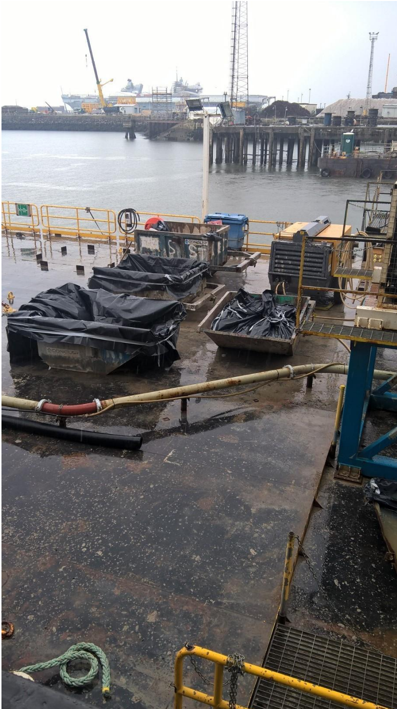
Figure 3 – Skips in place for controlled discharge
