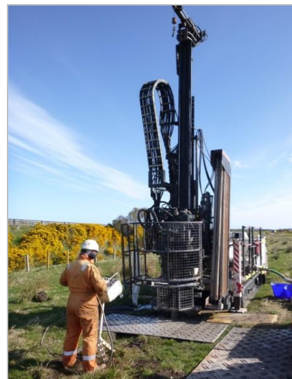
Ground investigation works for the scheme
