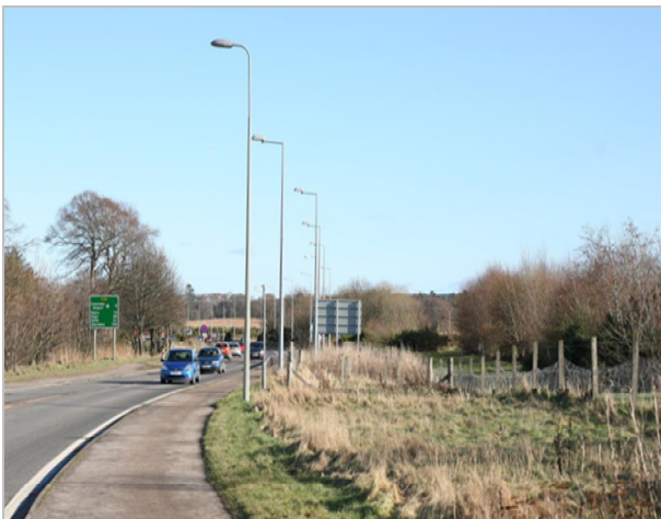
Existing single carriageway section of the A96 near Seafield
