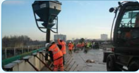
M74/M8 Link Viaduct Parapet
