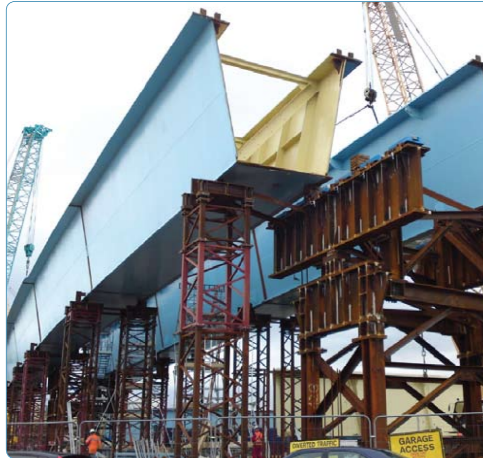
Launch steel at Stromness Street
