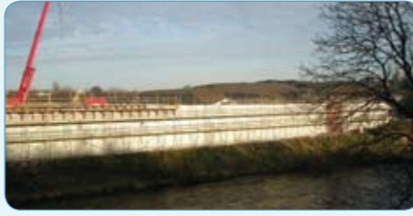
Auchenshuggle Bridge East Abutment
