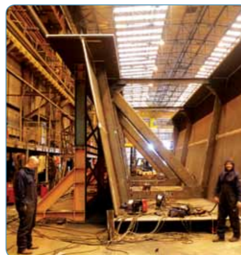
Beam Fabrication Shop
