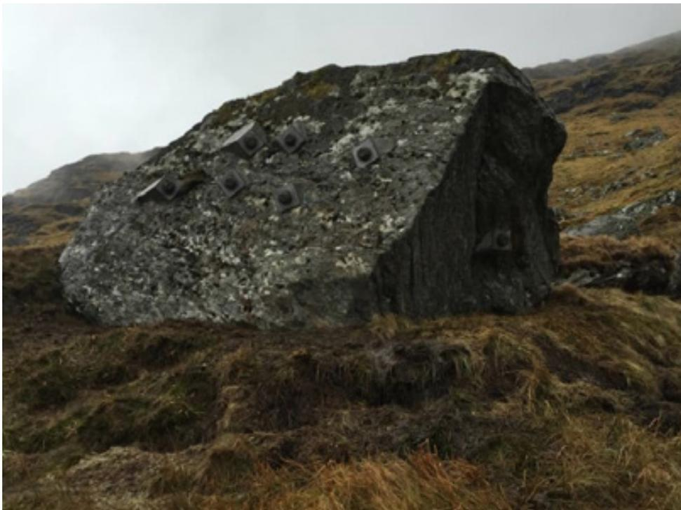
Figure 2.1 - Large boulder stabilised in situ on Beinn Luibhean
