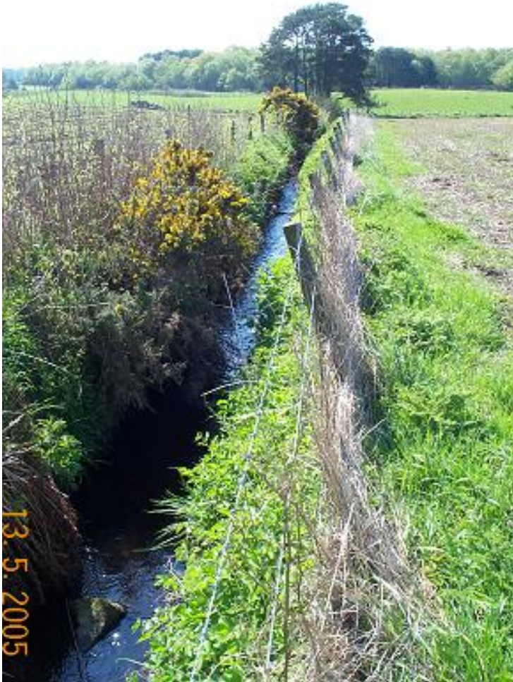
View looking upstream of Corsehill Burn in the location of the road. The channel is straight and deep which reflects past modification.
