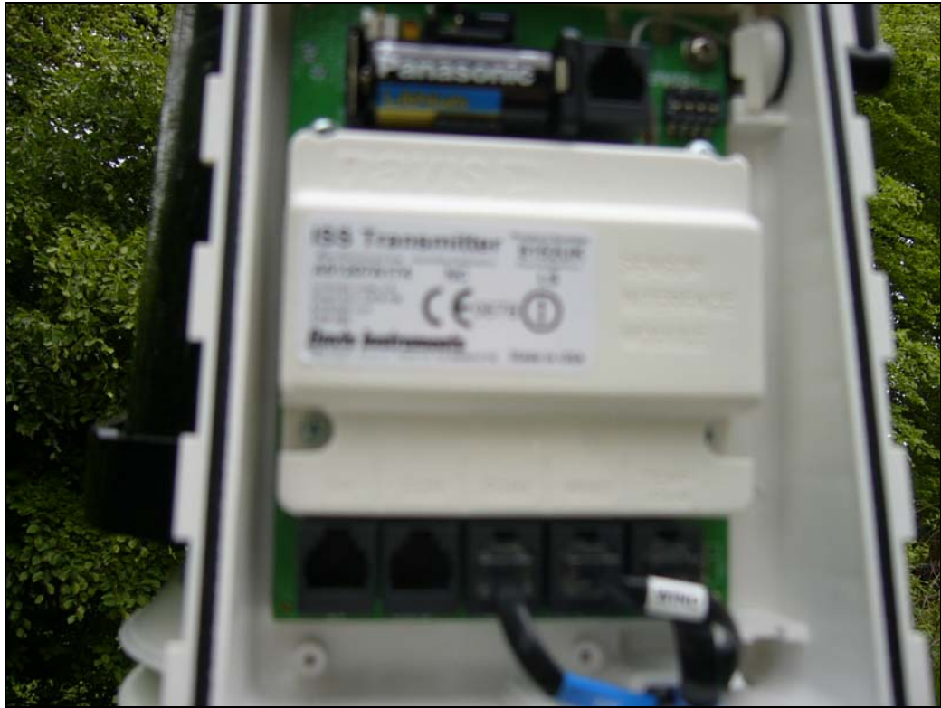
Figure 15. Cables removed but kept in position
