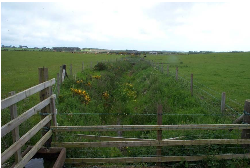
NO8707496024: View downstream. Straight ditch, no perceptible flow and filled with vegetation. Livestock fencing both sides.
