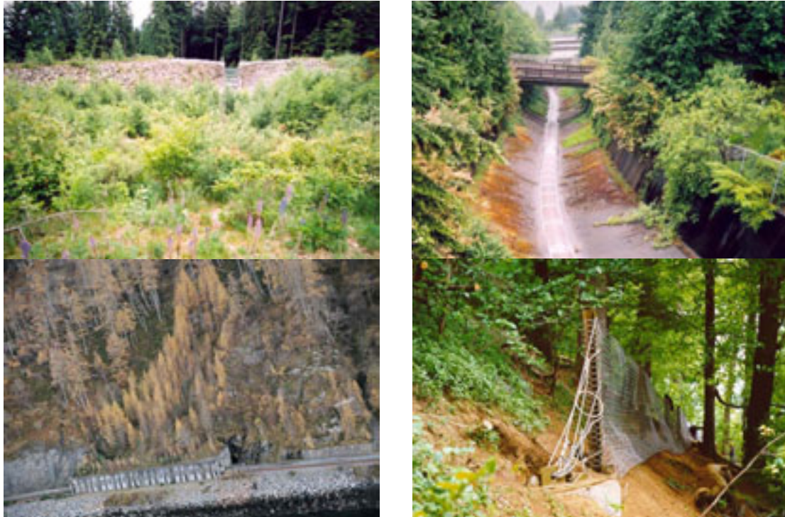
Examples of debris flow hazard reduction techniques. Top left: Debris basin. Top right: Lined debris channel. Bottom left: Debris shelter. Bottom right: Fence.
