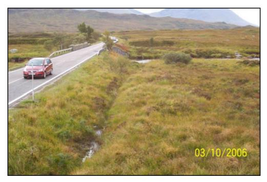
Figure 6.1 Road raised on embankment
