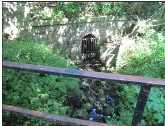
b) Downstream view of Woodside Burn at railway culvert inlet.
