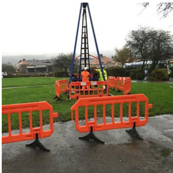
Ground investigation works
