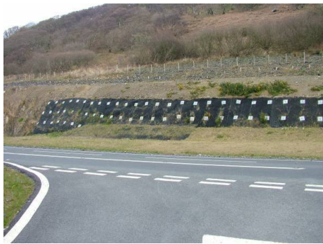
Figure 3: 1 YA Exposed macmatr and soil nailing
