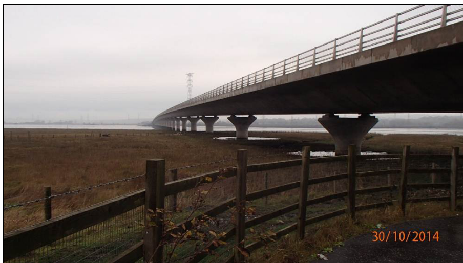
Figure A.11: Clackmannanshire Bridge viewed from the southern end
