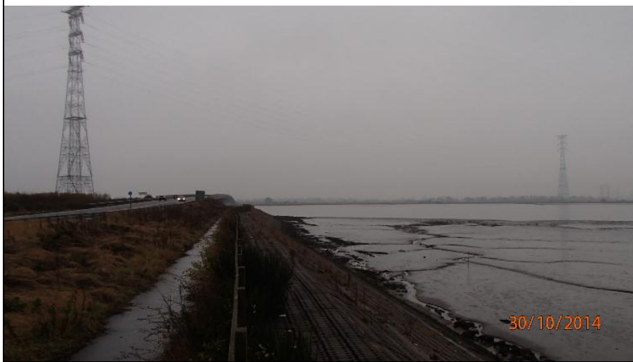
Figure A.8: Coastal realignment showing poor saltmarsh establishment at the toe of the embankment
