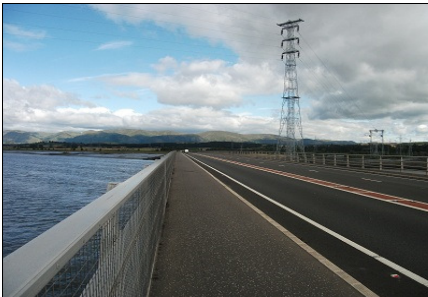
Figure 1.1: A876(T) Clackmannanshire Bridge looking north
