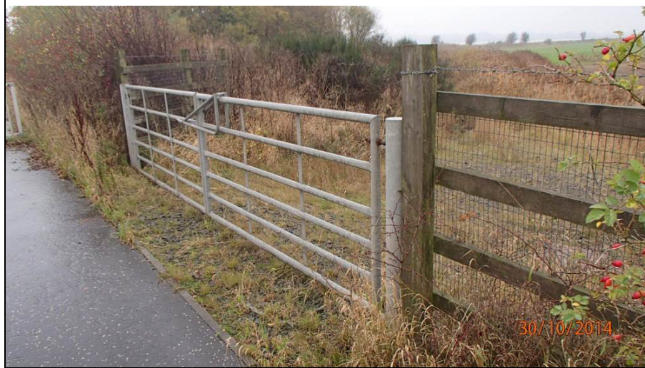
Figure A.10: Gap in the mammal fencing created by farm access gate
