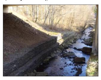
Photograph 4: Inchewan Burn (WF8) – downstream view of restored section underneath A9 bridge (typical example of a medium water feature).
