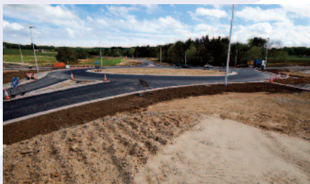
Goval East Roundabout
