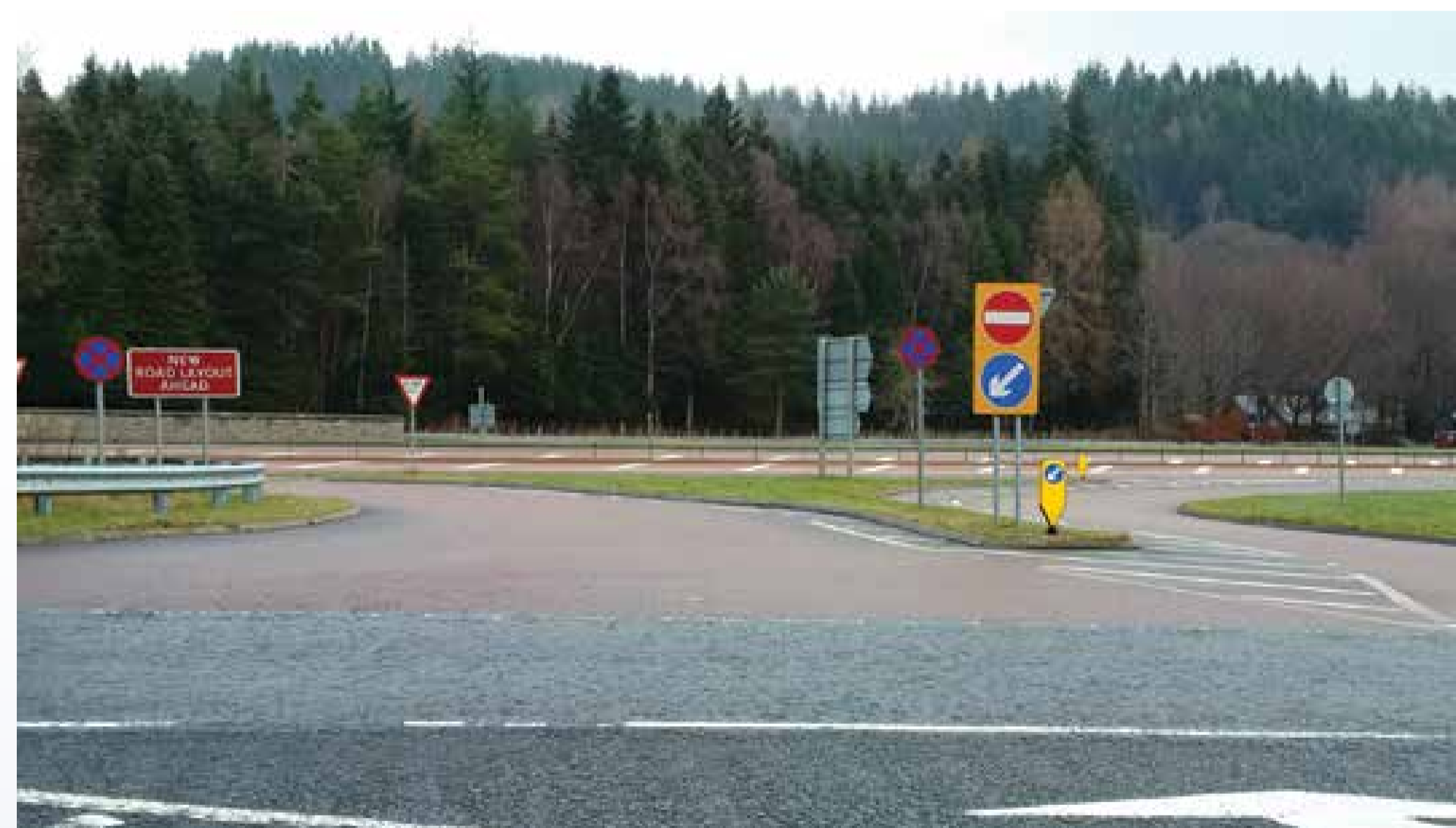
Pitlochry North junction
