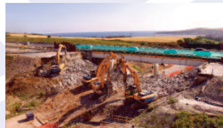
Demolition of A90 northbound at Stonehaven
