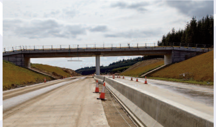
The wildlife bridge at Kirkhill
