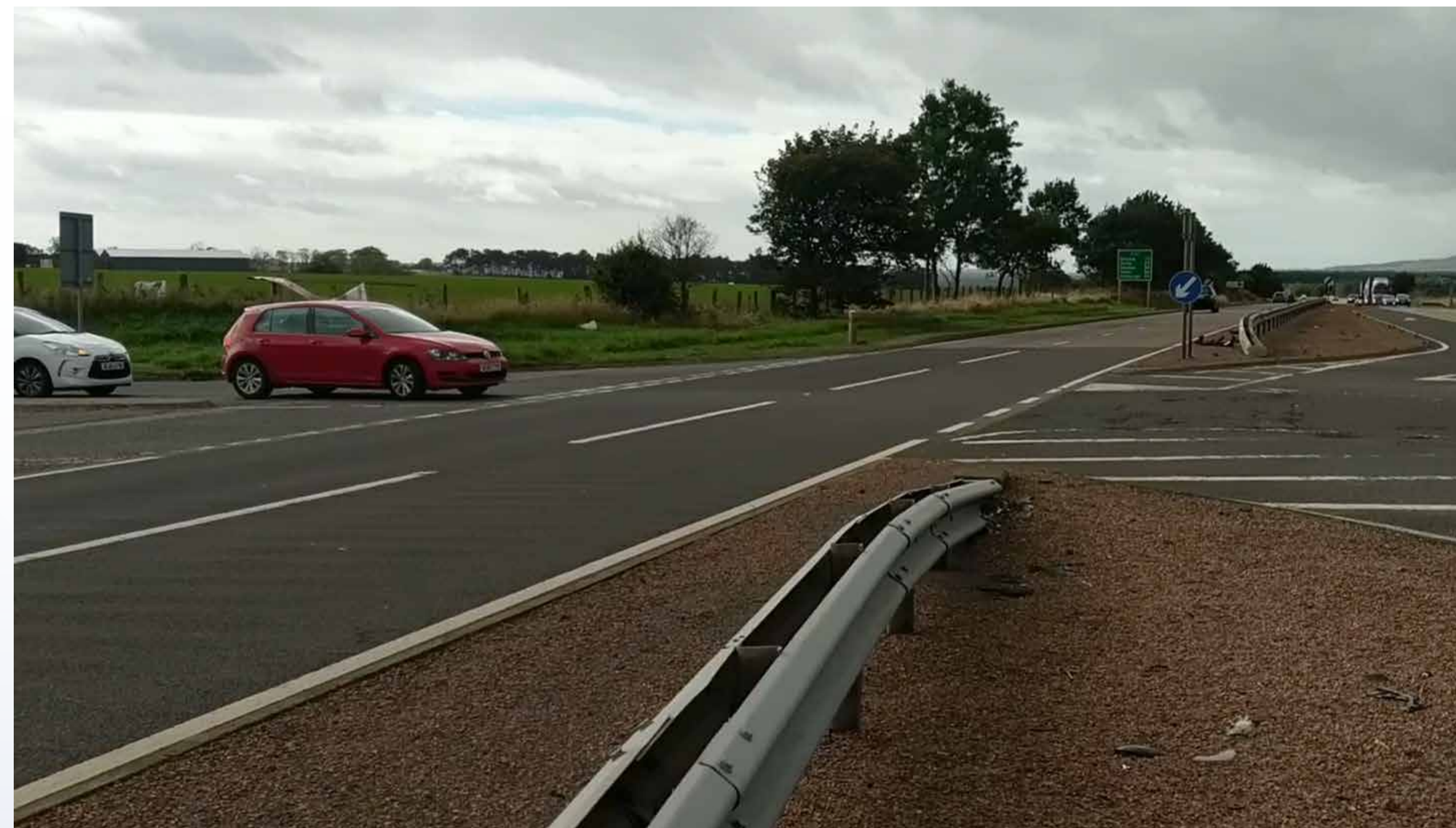
A90/A937 south junction looking south-west (southbound)
