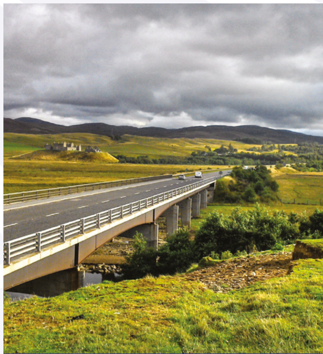
River Spey Bridge looking south
