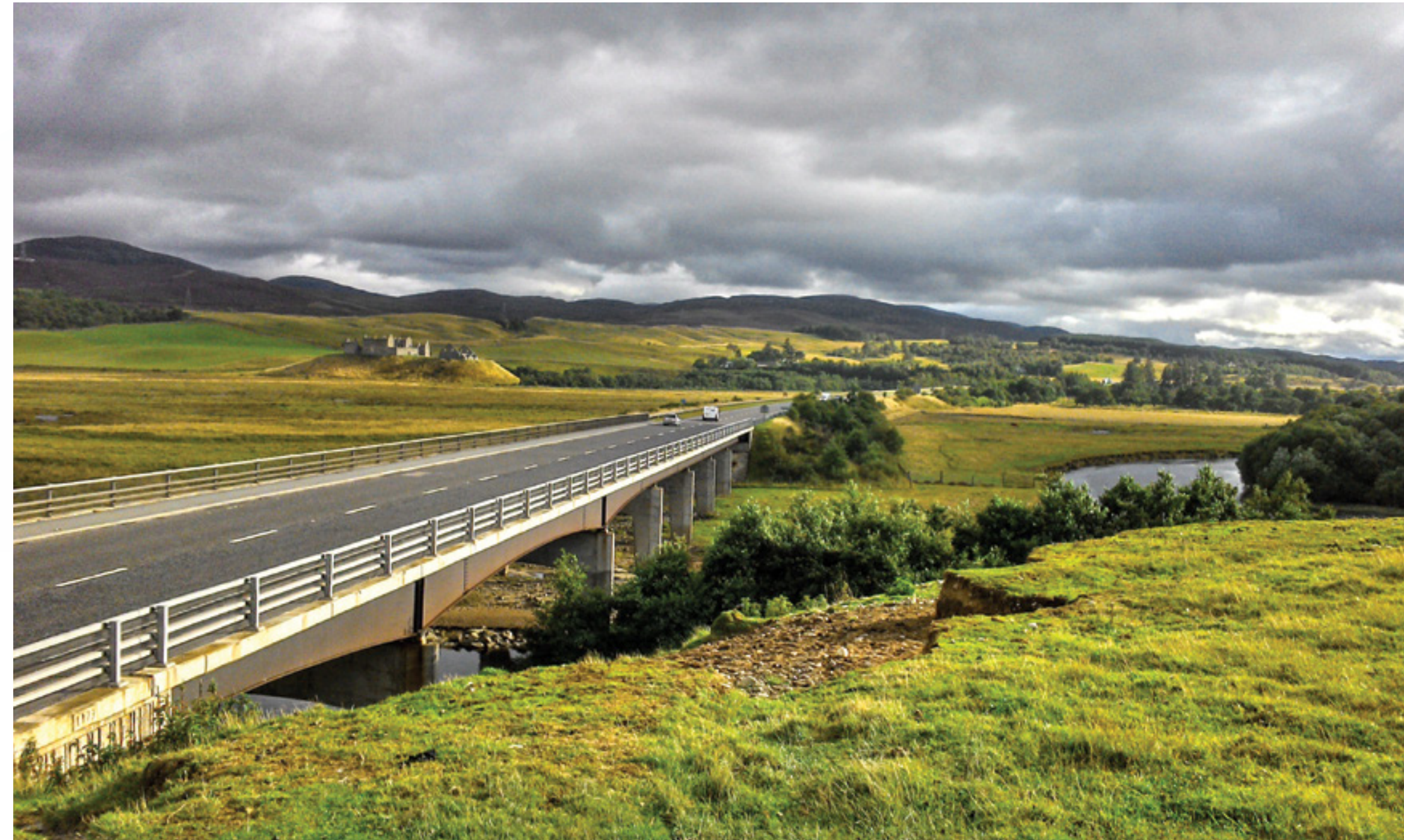
River Spey Bridge looking south
