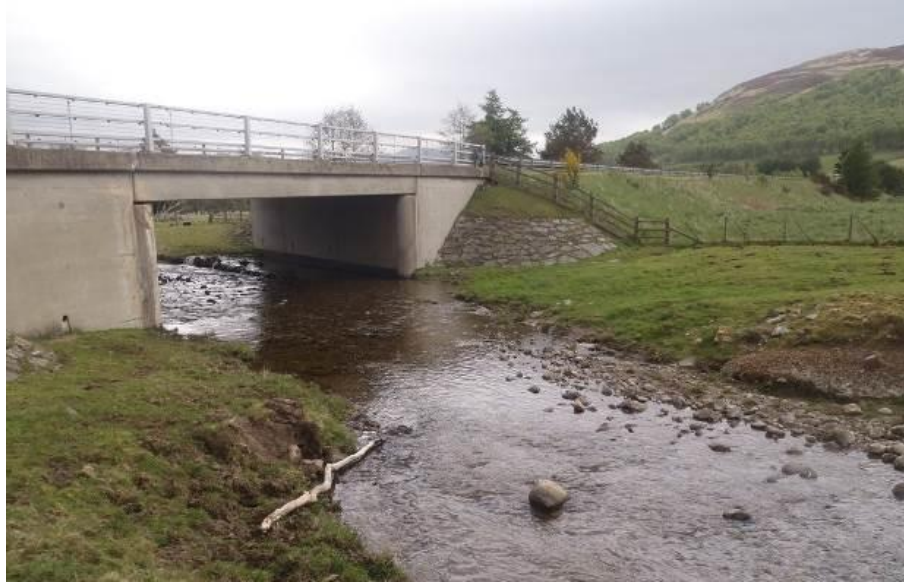
Photograph 7: Allt Bhaic – view downstream towards existing A9 crossing
