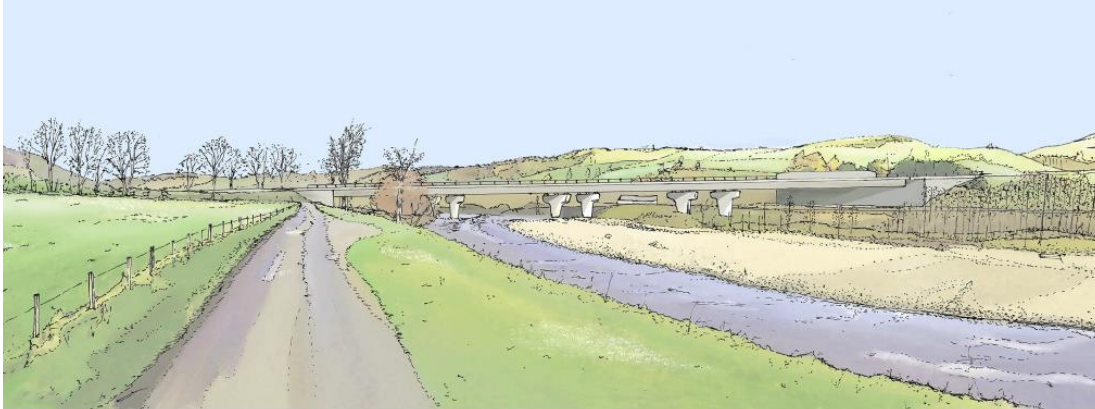
Illustration 4.1: Pier in the watercourse option for Essangal Underbridge (assessed as the proposed scheme)
