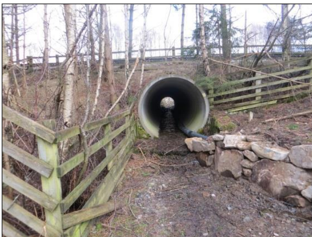
Photograph 5: Underpass east of WF134
