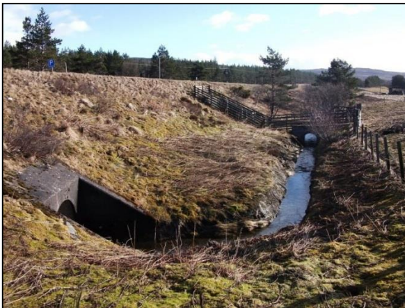
Existing A9 culvert - minor watercourse at WF159 looking downstream
