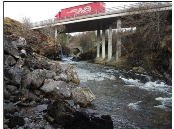
Existing Dalnamein Underbridge - principal tributary bridge crossing at WF158 looking upstream
