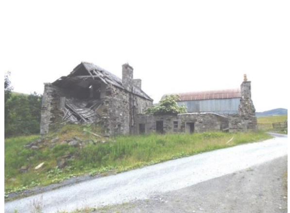
Photograph 6: General view on farmhouse from west
