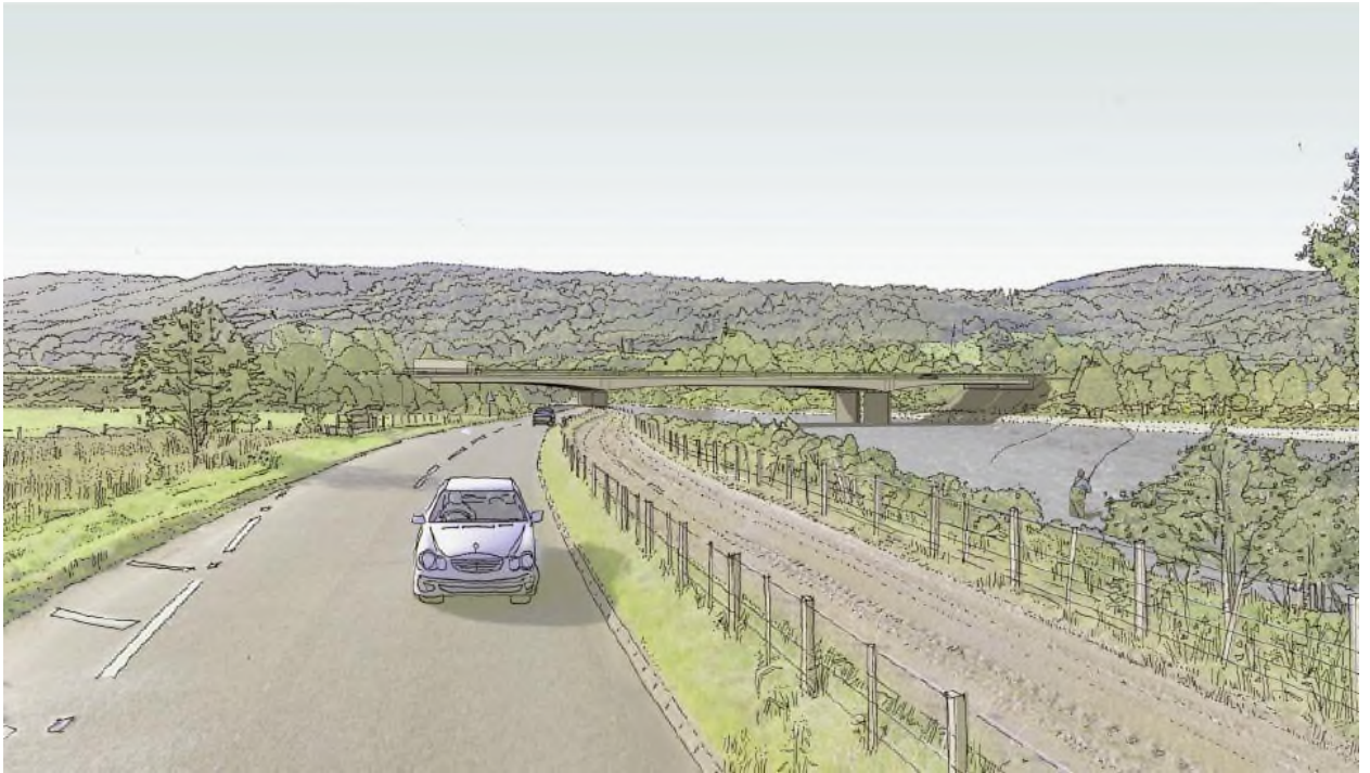
Illustration 4.3: Bowstring arch option (existing bridge retained) for Tummel Crossing (assessed as the proposed scheme)
