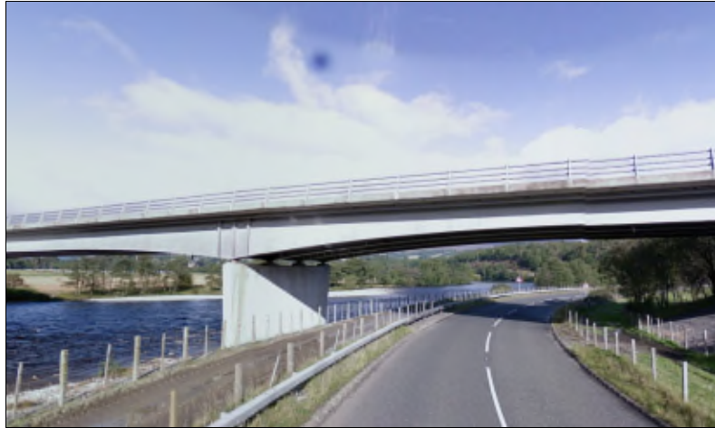
Image from Google Street View captured October 2008 © 2017 Google
