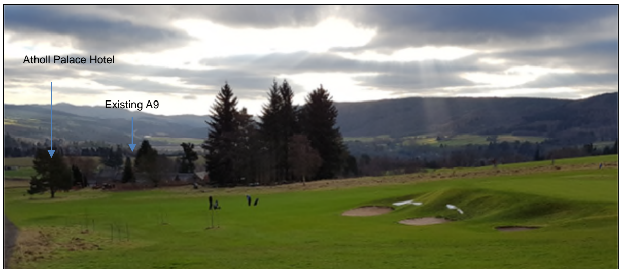
Photograph 14.21: Existing view looking south-east from the top of Pitlochry Golf Course towards the existing A9
