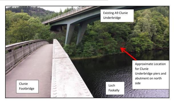
Photograph 1: Approximate location for piers and abutment for Clunie Underbridge on north side
