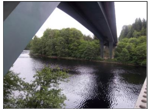
Existing Clunie Underbridge – looking south
