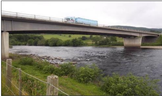
Existing Tummel Underbridge - looking south
