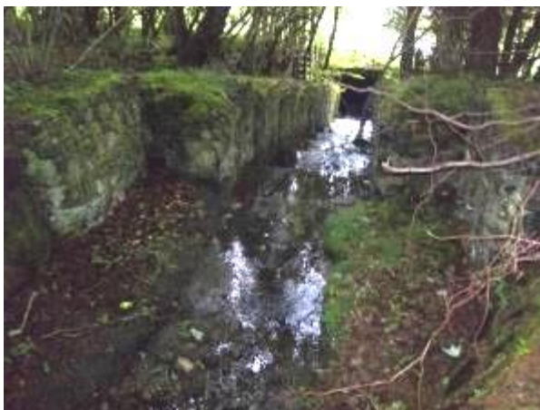
Photograph 5: View of WF65 downstream towards the existing A9 (stepped profile).
