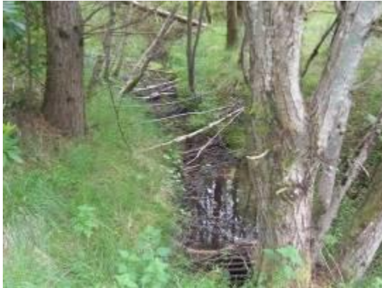
Photograph 13: View of WF74 upstream and modified section.
