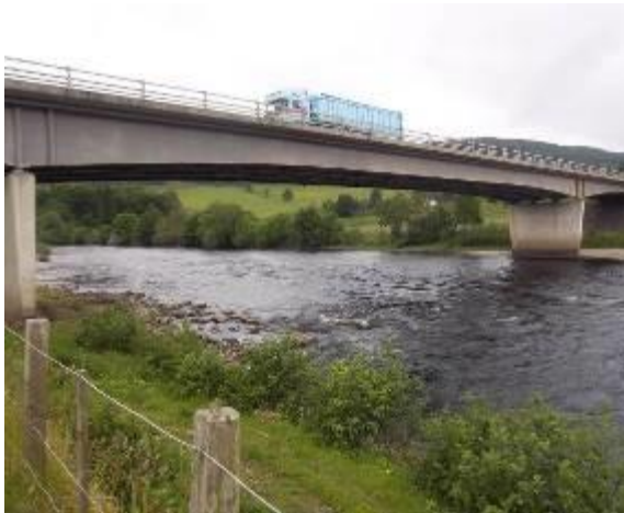
Photograph 17: Downstream view of WF70 (River Tummel) towards Tummel underbridge.
