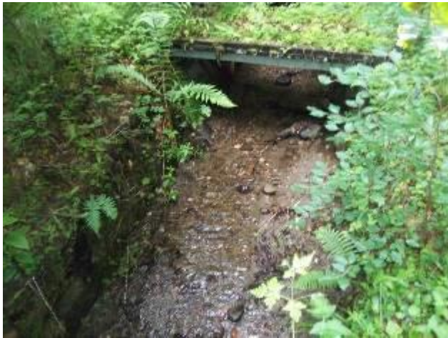
Photograph 15: View of WF76 (Allt an Aghastair) downstream towards existing A9 culvert.
