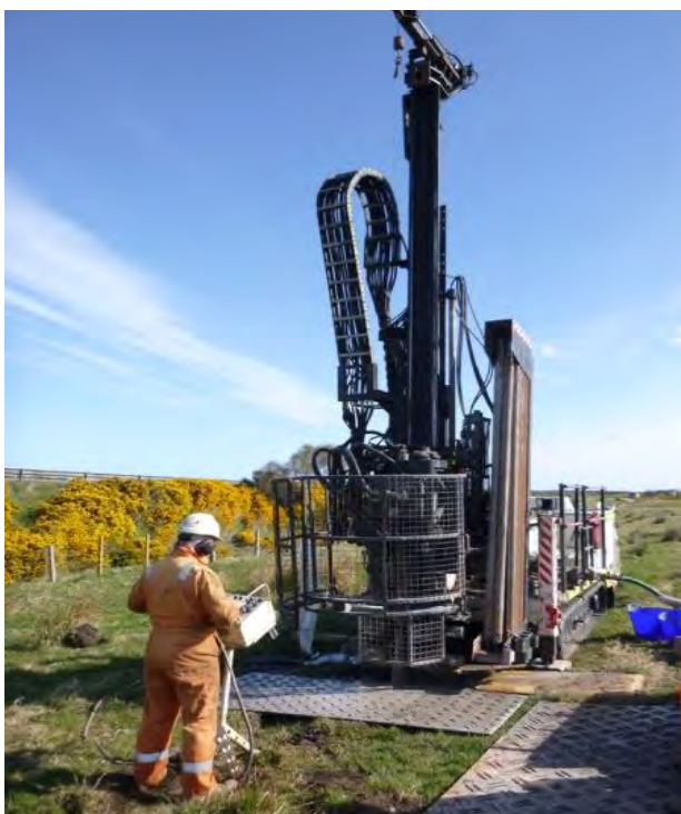
Photograph 12: Ground investigation works for the proposed scheme
