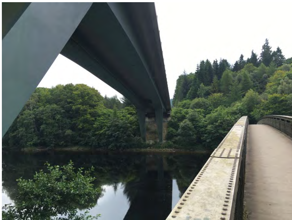
Photograph 4: Clunie Footbridge over Loch Faskally linking NMUs to crossing points
