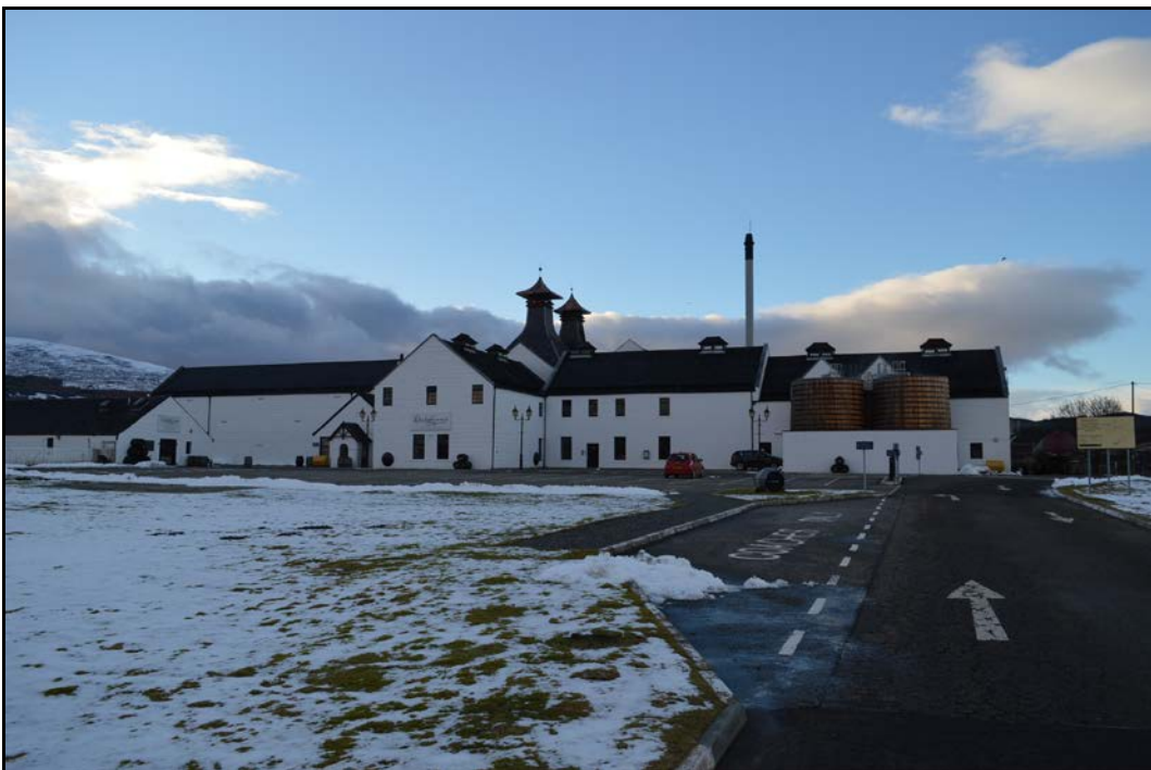
Photograph 8-2: Photograph of Dalwhinnie Distillery
