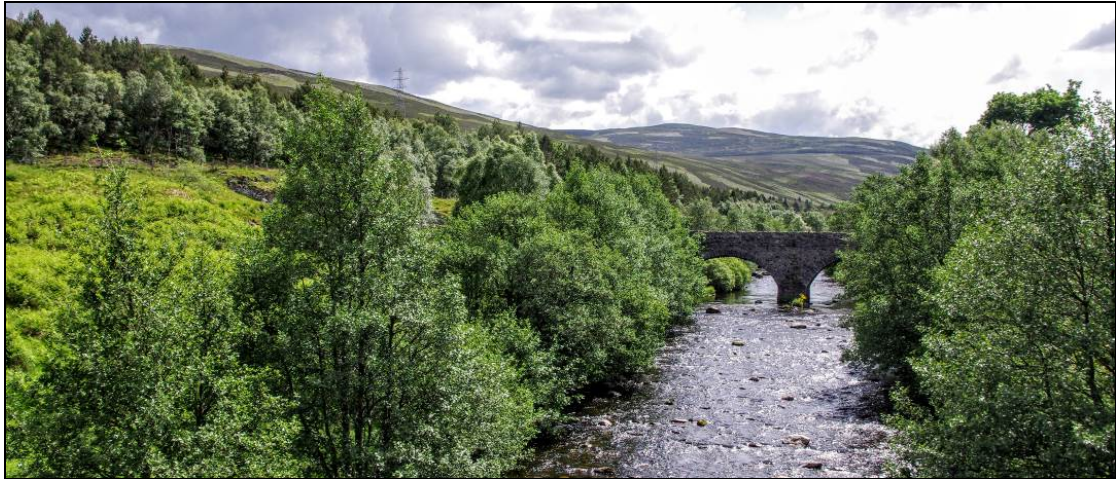
Photograph 15-3: Crubenmore Old Bridge (Asset 8.13), taken looking south from Crubenmore Bridge
