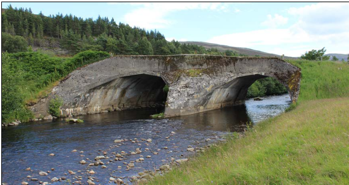
Photograph 15-4: Crubenmore New Bridge (Asset 8.14), taken looking north
