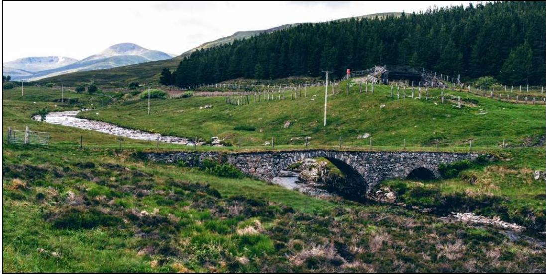
Photograph 15-1: Wade Bridge (Asset 8.3) looking south
