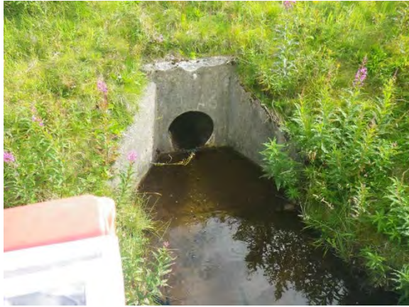
Photograph 11.4.3.22 – Downstream exit of pipe crossing
