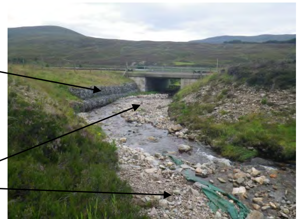
Photograph 11.4.3.37 - Downstream to crossing
