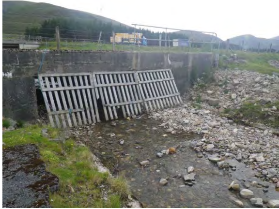
Photograph 11.4.3.5- Downstream to crossing
