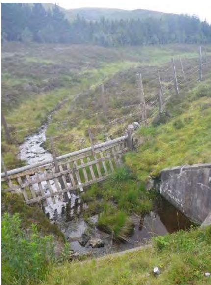
Photograph 11.4.3.10- Upstream of crossing, confined channel
