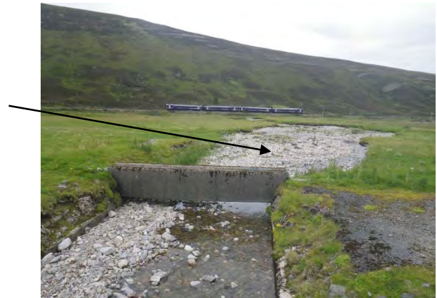
Photograph 11.4.3.4- Unknown structure crossing downstream
