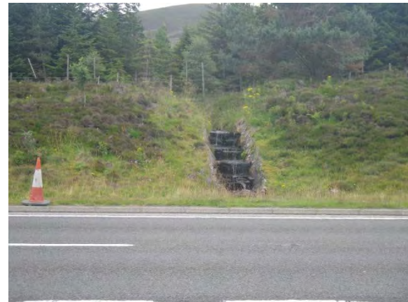
Photograph 11.4.3.26 – Looking upstream- Stepped cascade into crossing
