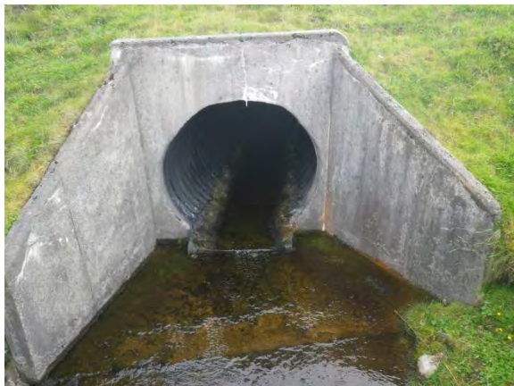
Photograph 11.4.3.8- Upstream to pipe
