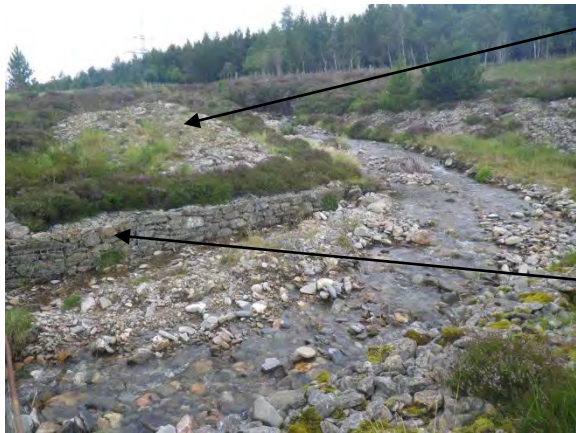
Photograph 11.4.3.15-Upstream bank protection
