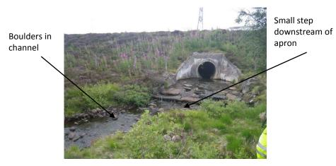
Photograph 11.4.3.38 - No deposition in culvert
