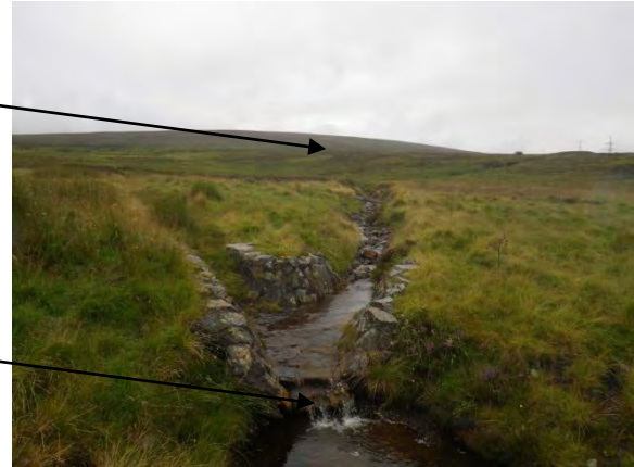
Photograph 11.4.3.66- Upstream to channel realignment creating a step in bed
