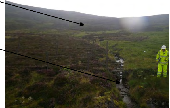
Photograph 11.4.3.102 – Upstream of crossing
