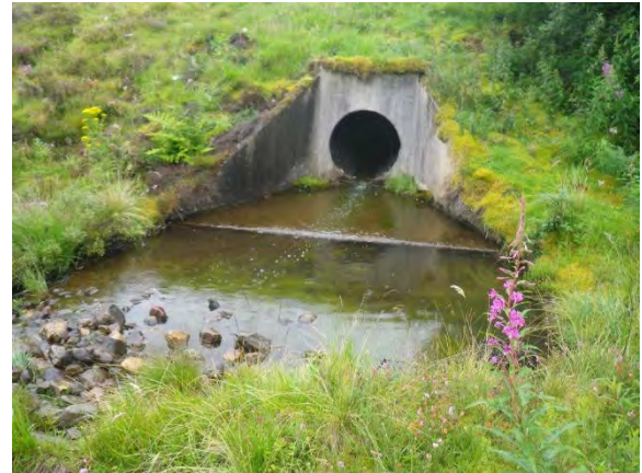
Photograph 11.4.3.72 - Crossing exit- Over wide, shallow channel
