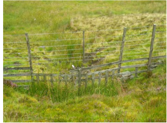
Photograph 11.4.3.90 -Downstream crossing exit
