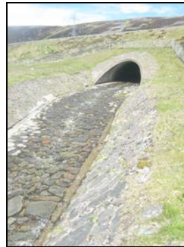
b) Downstream view west of A9 showing bed protection
