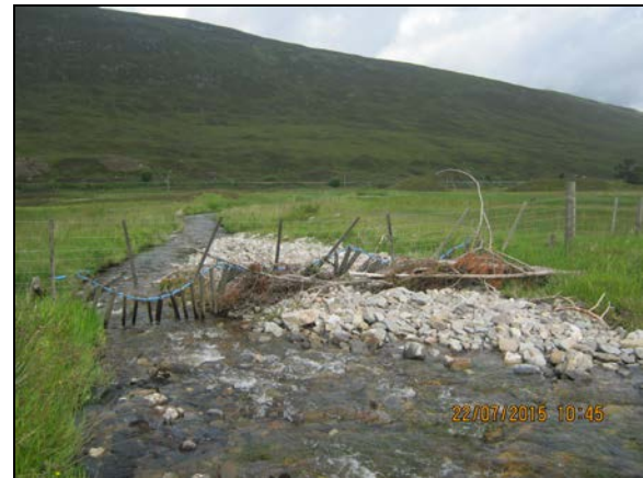
b) Downstream view west of A9, showing areas of deposition
