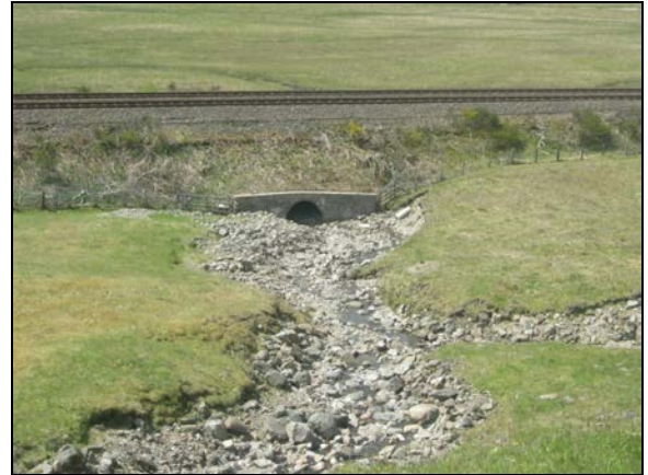
b) Downstream view west of A9 showing evidence of lateral channel migration
