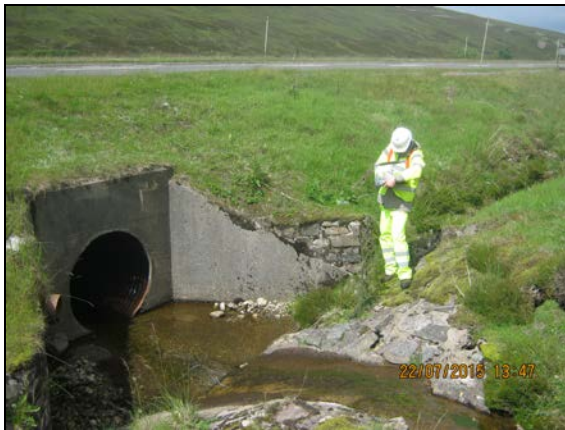
a) Upstream view east of A9, showing bank protection
