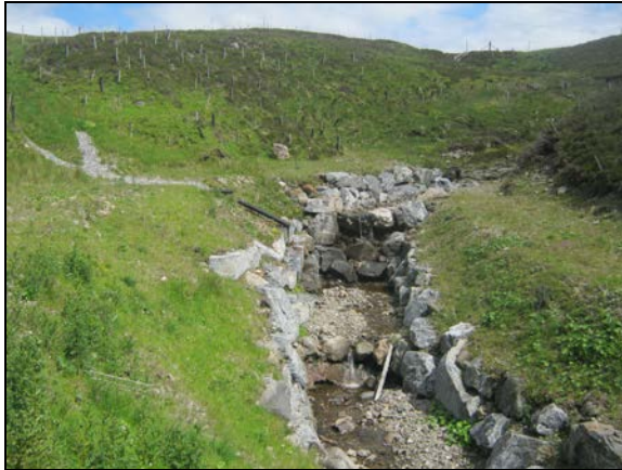
a) Upstream view east of A9, showing evidence of bank protection
