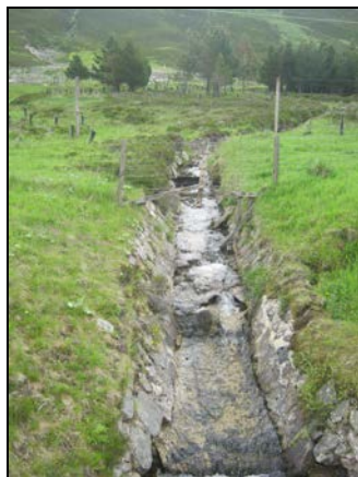
Photograph 11-8: Allt an Creagach (Hydro ID 31/ MW 7.11)
