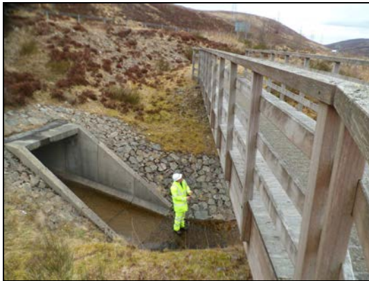
a) Downstream view west of A9
