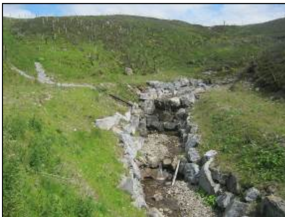
a) Upstream view east of A9, showing evidence of bank protection
