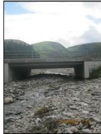
b) Downstream view west of A9, showing pinch-point to sediment movement
