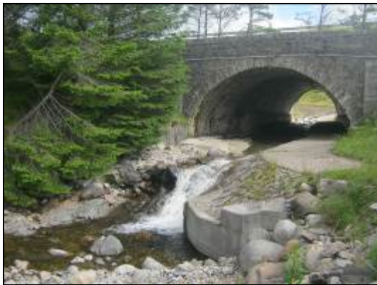
a) Downstream view of channel modifications west of A9
