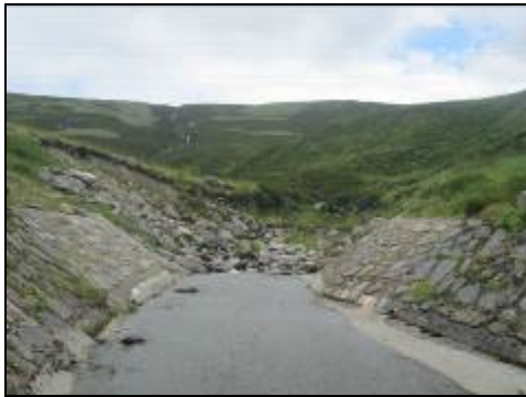
a) Upstream view east of the A9, showing bed and bank protection
