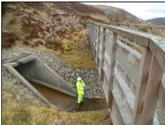
a) Downstream view west of A9
