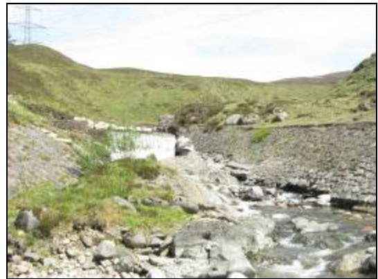
b) Upstream view of the Hydro Scheme east of A9
