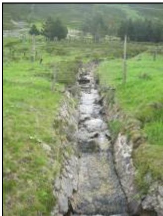
a) Upstream view east of A9, showing evidence of bed protection b) Downstream view west of A9
