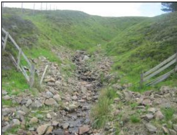
a) Upstream view east of A9, showing evidence of deposition
