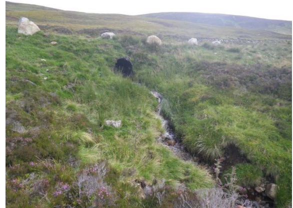
Photograph 11.4.3.37- Pipe under track
