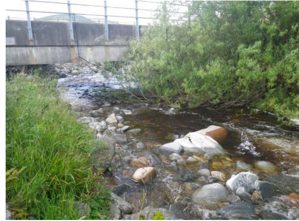
Photograph 11.4.3.17 downstream to railway crossing
