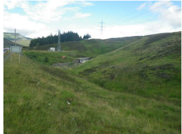
Photograph 11.4.3.15 -Drainage into crossing 2
