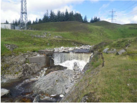
Photograph 11.4.3.8 -Weir upstream of crossing
