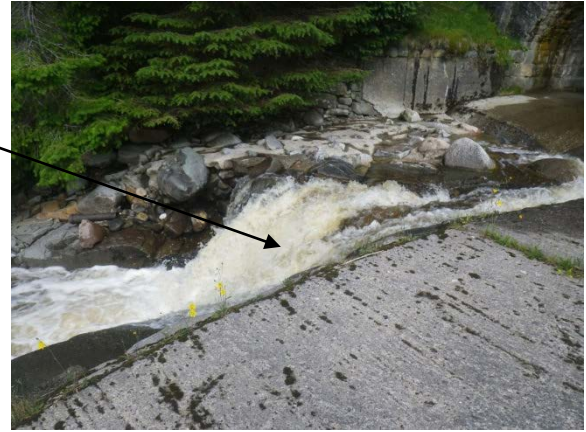
Photograph 11.4.3.5-Scour creating step in bed downstream of crossing
