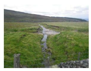
Photograph 11.4.3.95- Downstream to confluence with crossing 64, failing channel banks
