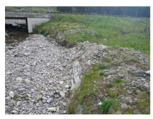
Photograph 11.4.3.88- Erosion of right bank
