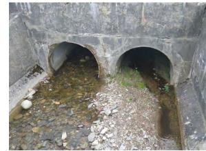
Photograph 11.4.3.98- Deposition in both pipes downstream of crossing
