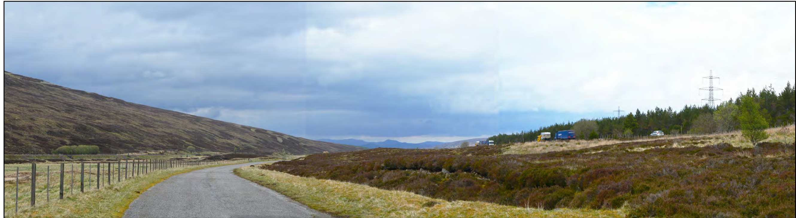
VIEW LOOKING NORTH PARALLEL TO THE A9 FROM NCN7 NORTH OF DRUMOCHTER LODGE
