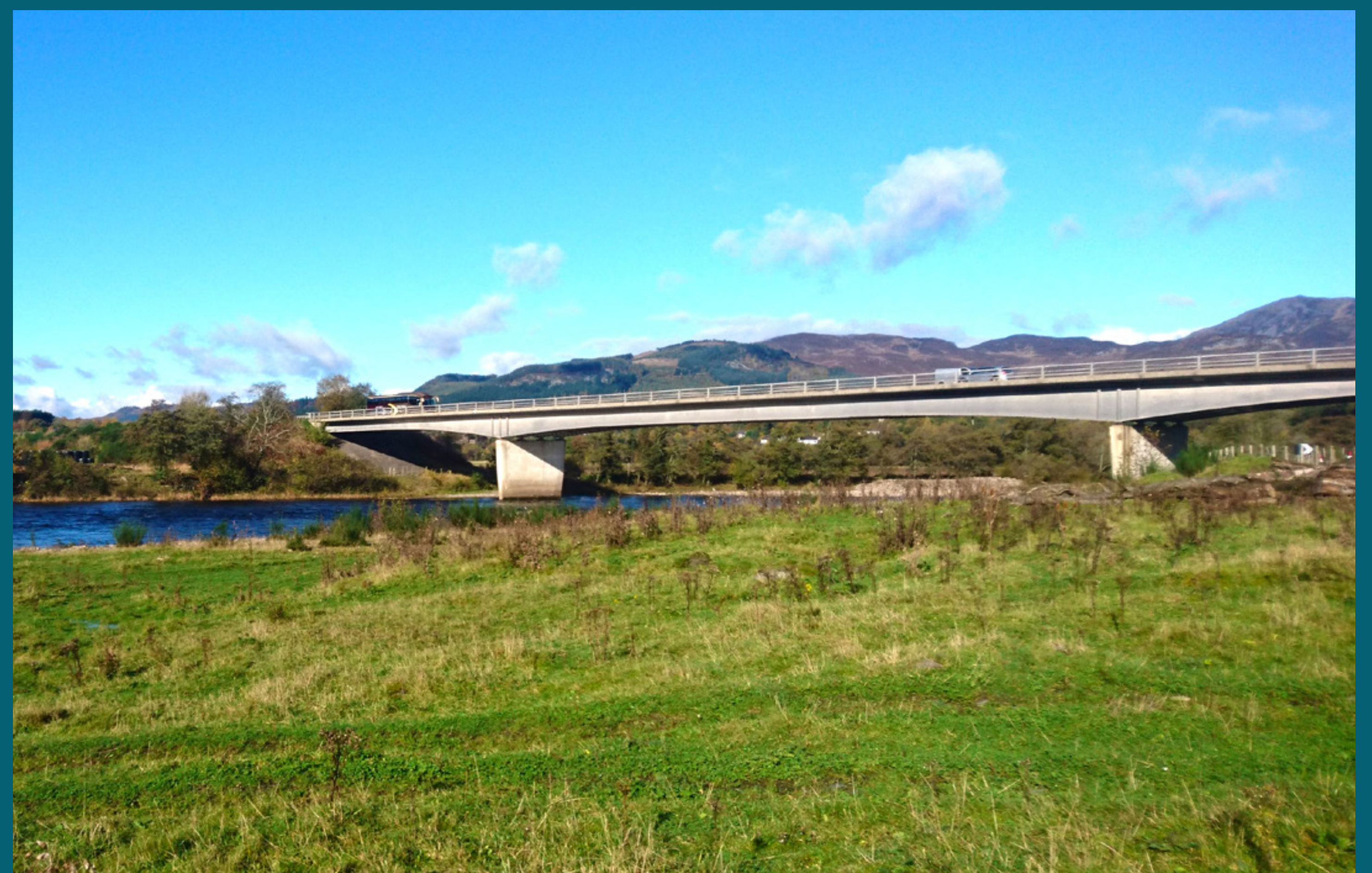
View of existing River Tummel crossing
