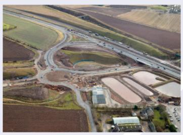
**Stonehaven:** The new B979 Netherley Road Overbridge is complete and a new roundabout for the Fastlink is almost finished.
