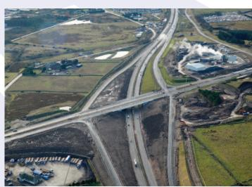
Charleston Junction: The former A956 bridge has been replaced with a new structure taking the AWPR over the A90.
