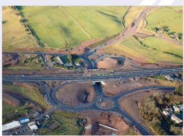
Balmedie Underpass: The new underpass can be clearly seen with the new roundabouts and access roads approaching completion.
